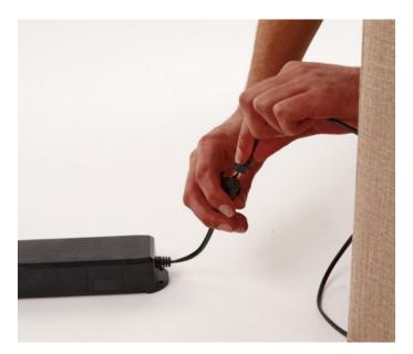
7. Connect the power cable to the transformer and mains plug.
